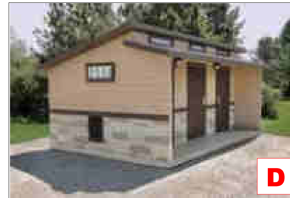
PRE-FAB RESTROOM BUILDING W/STORAGE
