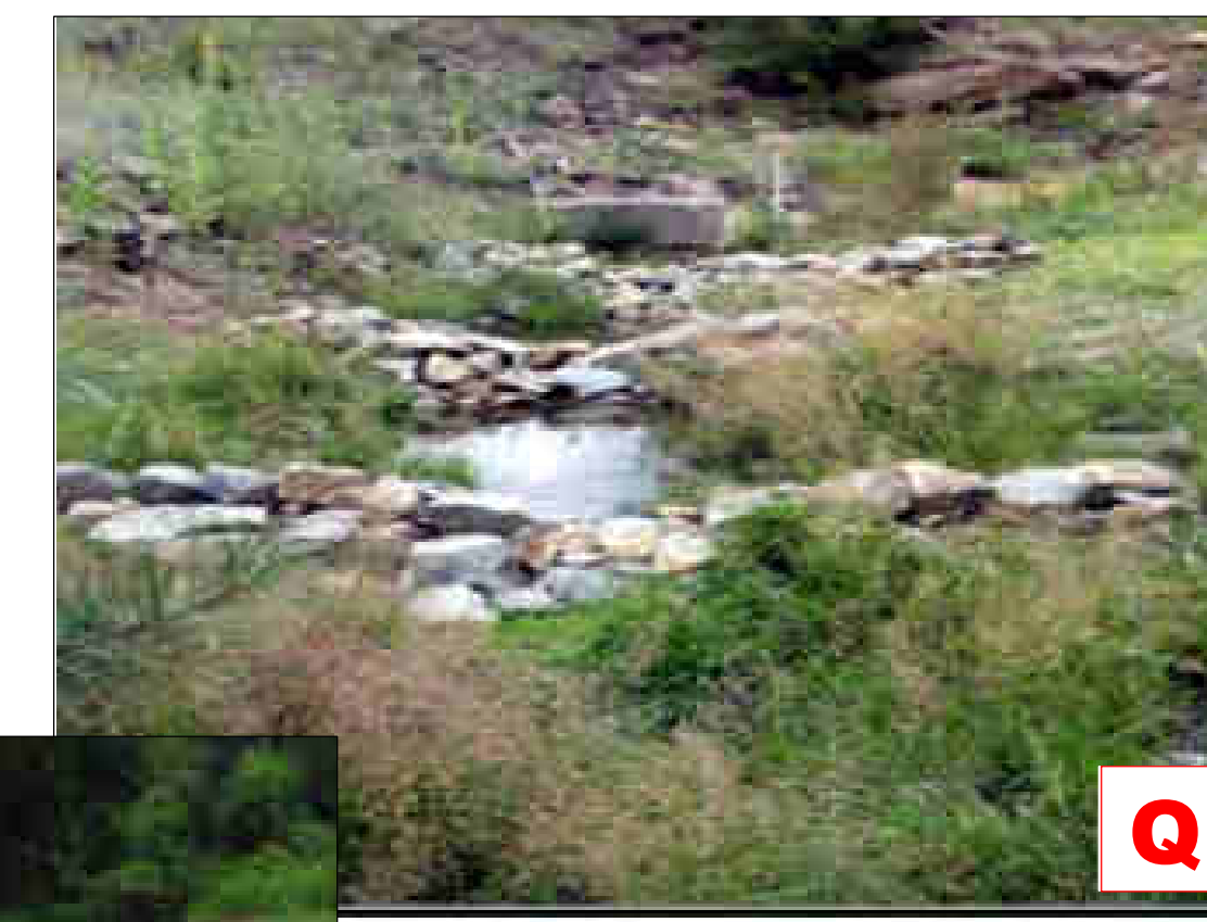
ROCK CHECK DAMS
