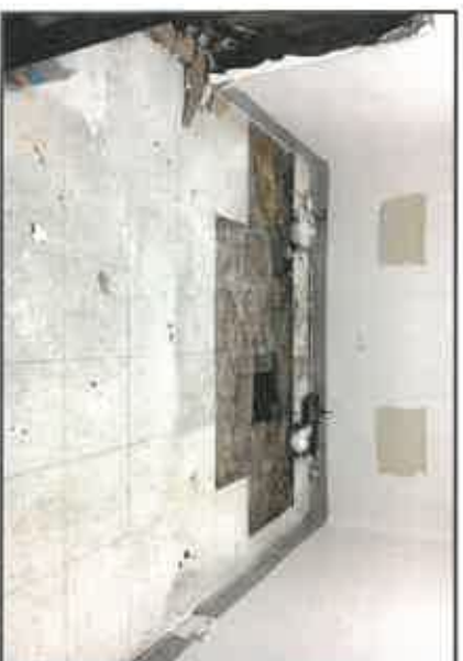
06.01 MAINTENANCE OF WOOD, PLASTICS & COMPOSITES Rotted Raised Floor
