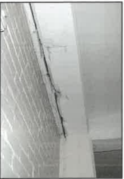
04.20 NORTH WALL GAP AT FLOOR BEAM
