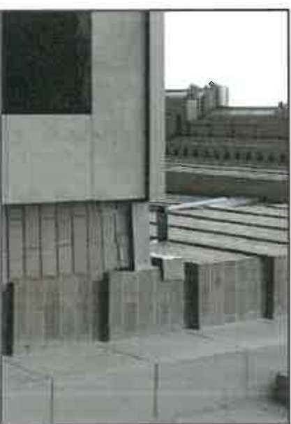
04.03 LOOSE BRICK AT GARAGE Overload Condition
