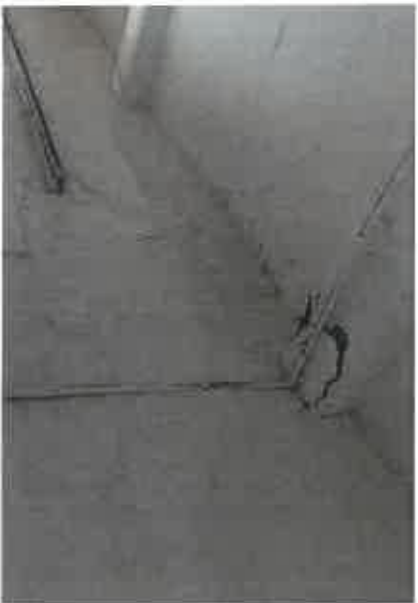
03.00 CONCRETE Spalled Beam
