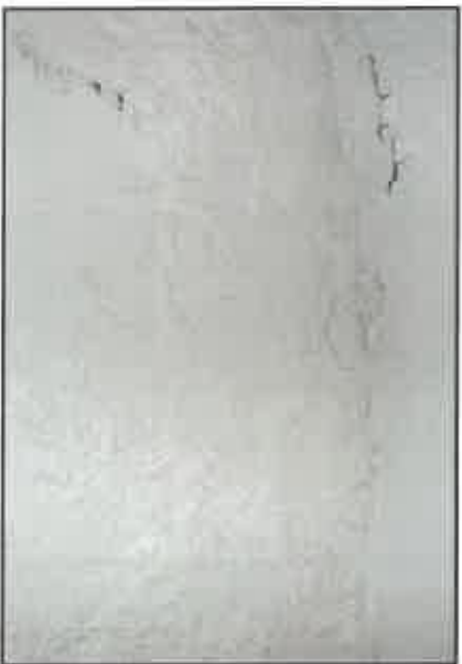
04.03 BUBBLED PAINT FROM MOISTURE INFILTRATION
