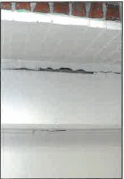
04.20 NORTH WALL SEPARATION AT COLUMN
