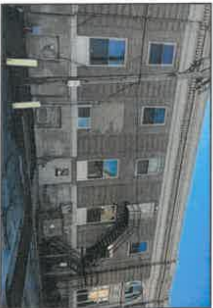
08.16 WALL VENTS Inconsistent Size and Finish
