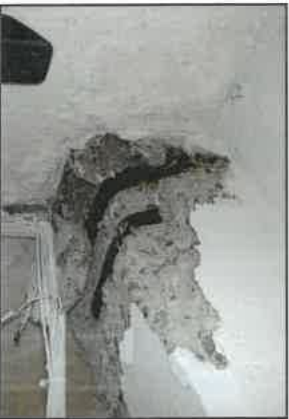
03.03 SPALLED CONCRETE AT ROOF BEAM
