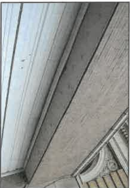
05.12 STEEL LINTEL AT GARAGE DOOR
