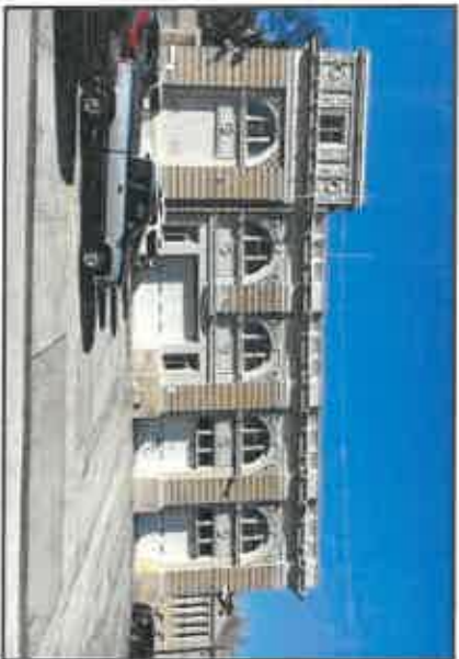
04.08 MASONRY INFILL Modified Openings
